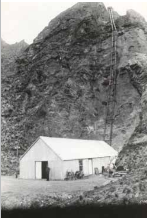
Dynamo Shed, Bullendale
