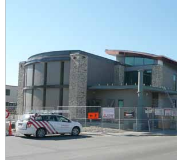
Construction at 190 Waenga Drive is underway
